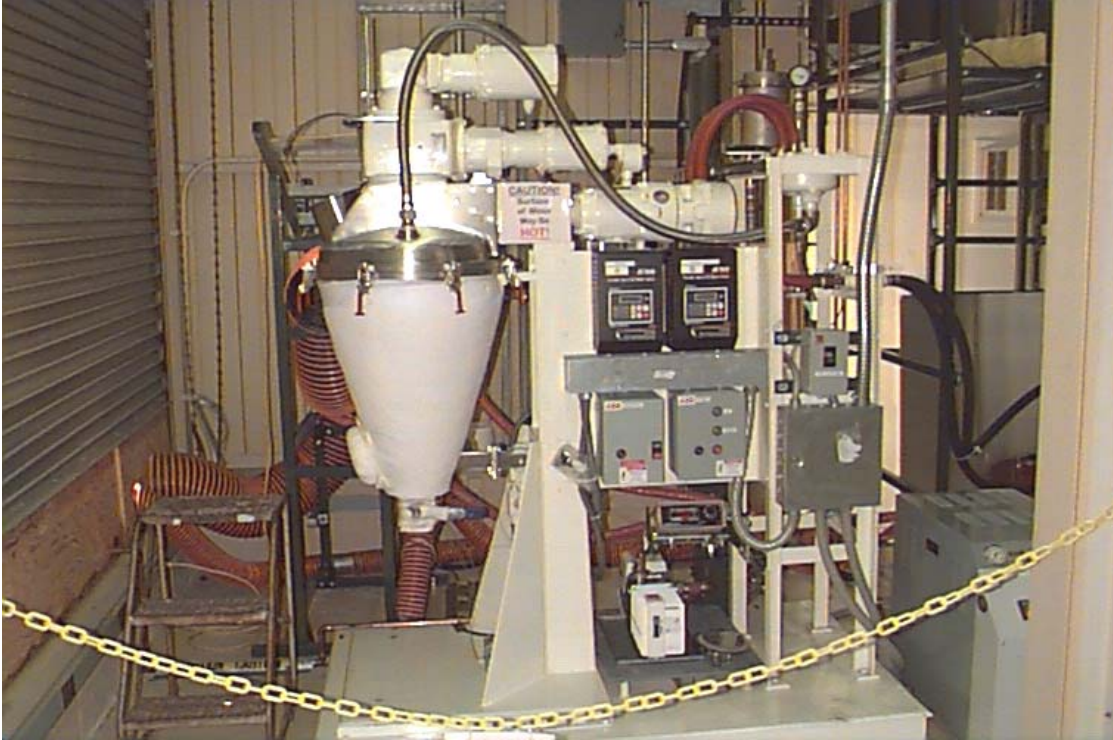
Fig. 3.1. SPSS mixer and process controls.
