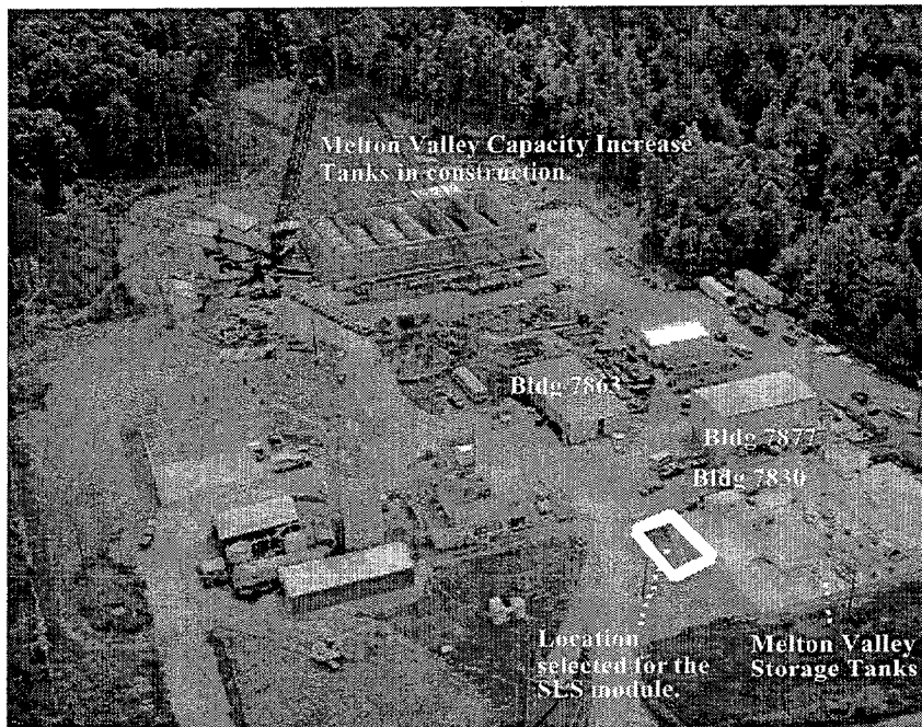
Fig. 2. Aerial photograph of the MVST facilities during construction for the capacity increase tanks.
