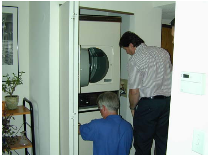
Figure 2.4 Phase I Instrumentation Installation
