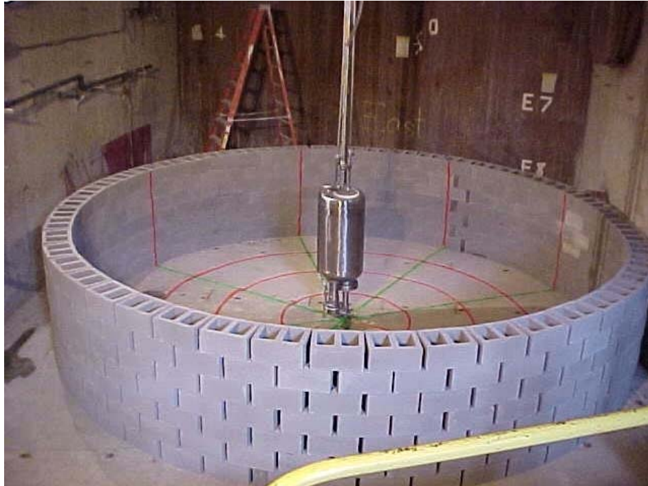
Fig. 13. Mock tank in TTCTF before addition of plastic liner.
