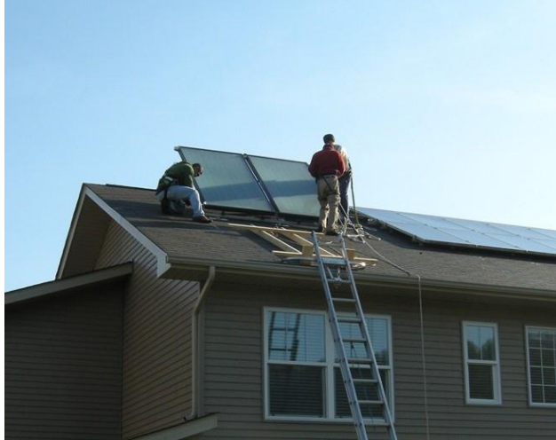
Fig. 3. Sustainable Future removes solar thermal panels at CC3.
