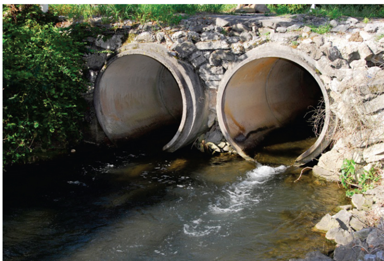
Fig. 4.46. Contaminated storm sewers were the primary source of mercury contamination in Poplar Creek.
