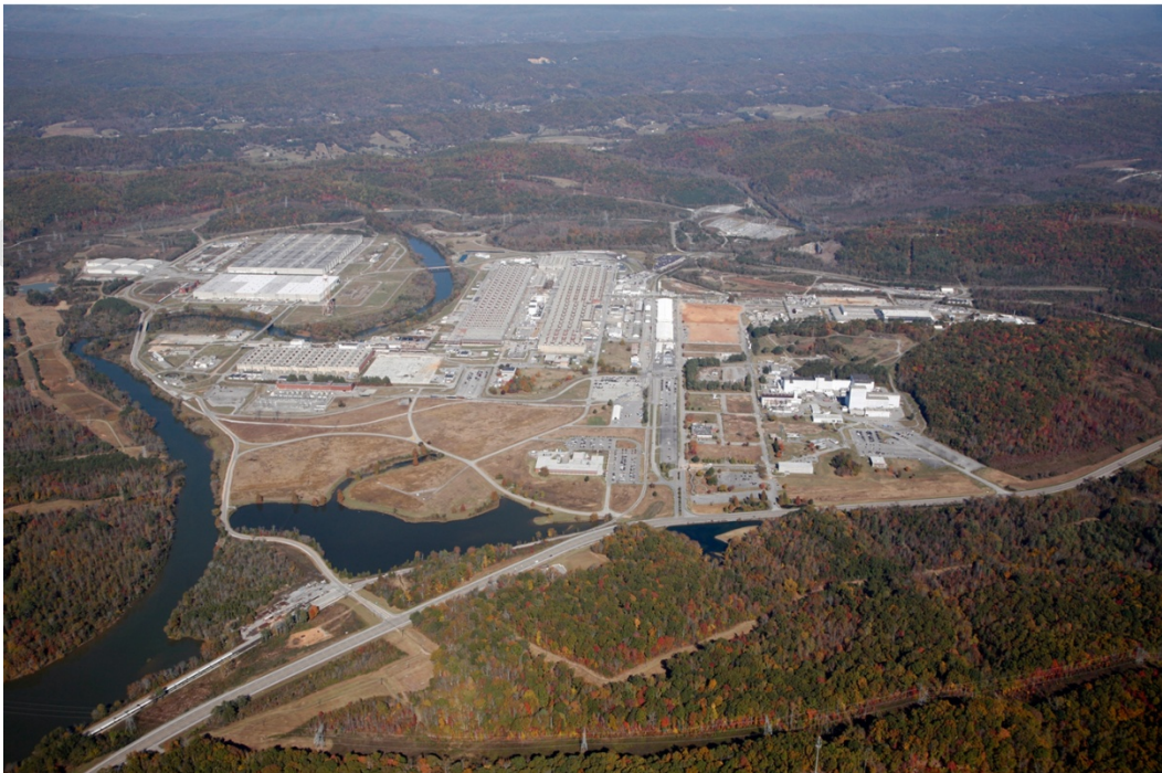
Fig. 1.9. East Tennessee Technology Park.
