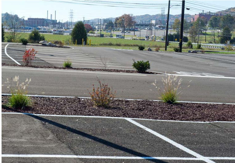
Fig. 4.15. Permeable pavement and native plantings contribute to Energy Independence and Security Act Section 438 requirements. (Source: Kathy Fahey, Y-12 Photography)
