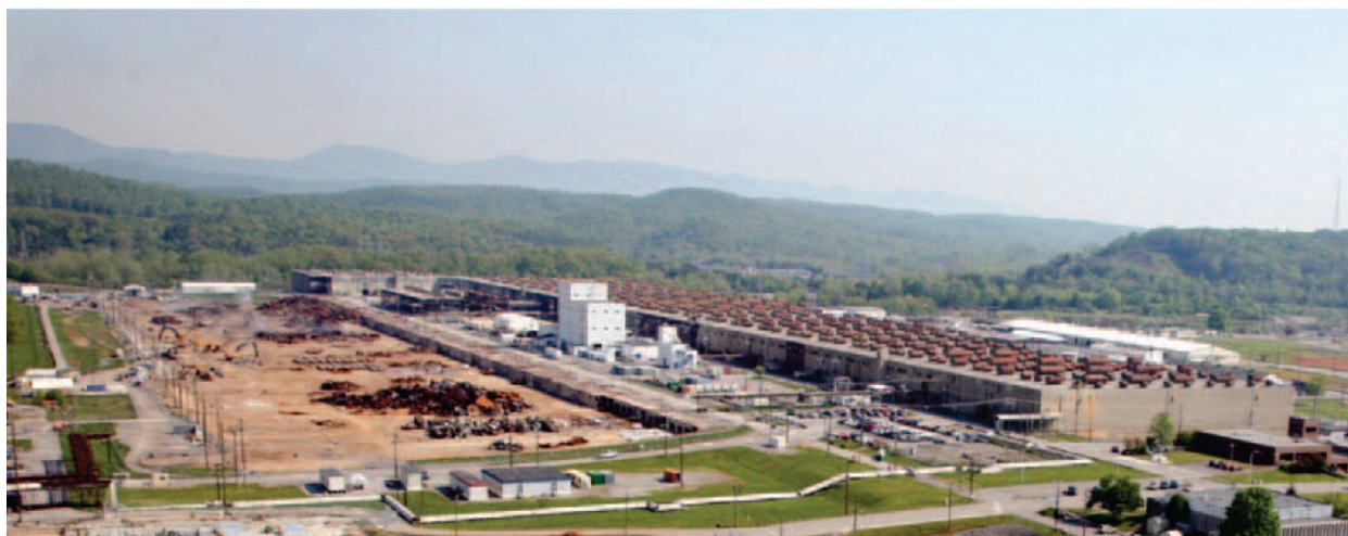
Fig. 3.63. Building K-25 after demolition of the west wing.
