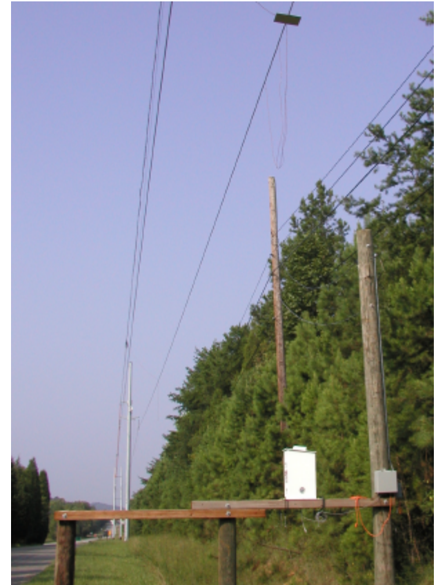
Laser at mid-span measure conductor sag
