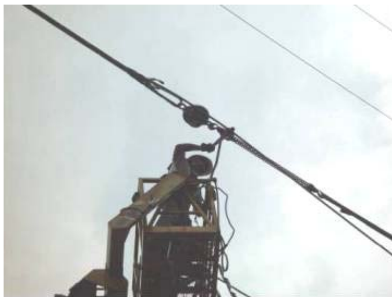
Figure 4- Sagging with chain hoist and dynamometer
