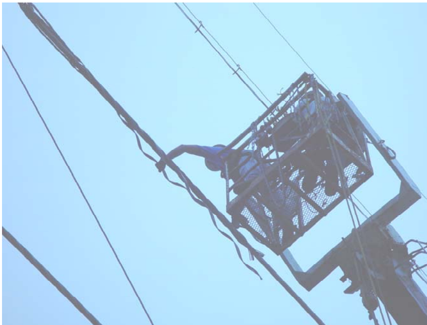
Figure 4- Installation of PLP THERMOLIGHT™ DEAD ENDS next to stringing chain
