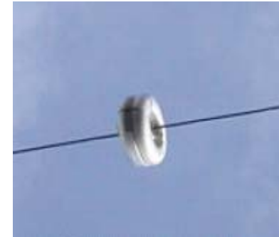
Wireless Communication to Ground Station
