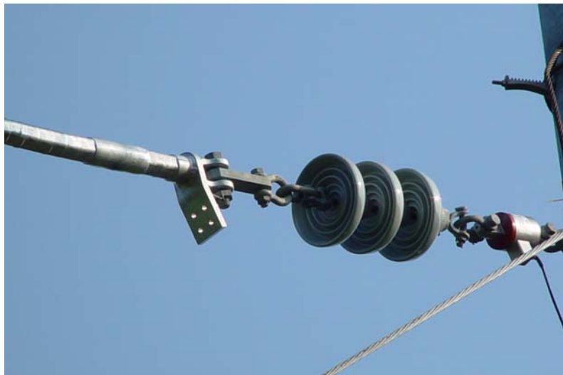
Figure 5- Installed Alcoa compression dead end next to insulator and dead end tower
