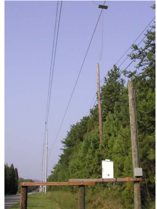
Laser at mid-span measure conductor sag
