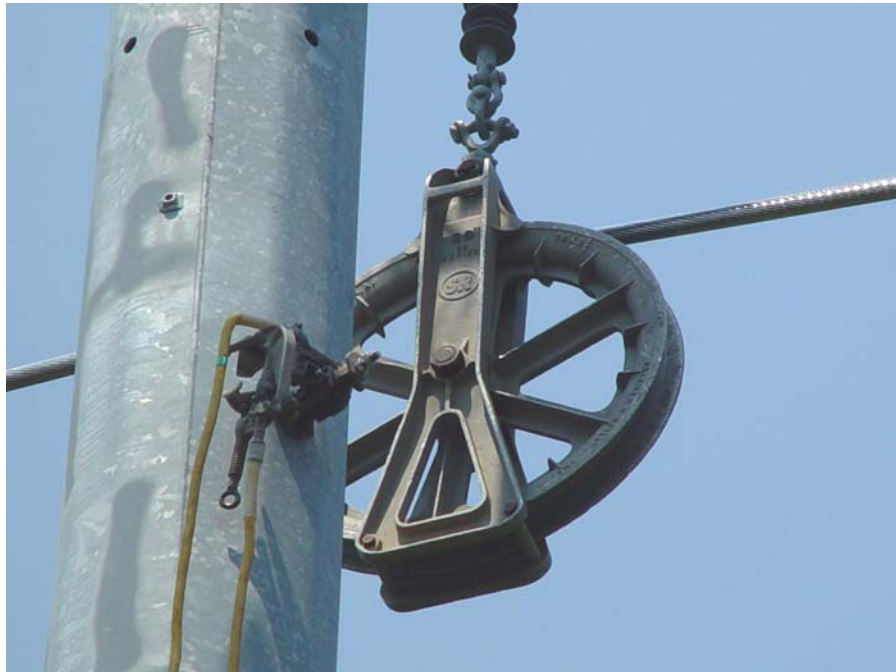
Figure 2- Sheave used in the installation
