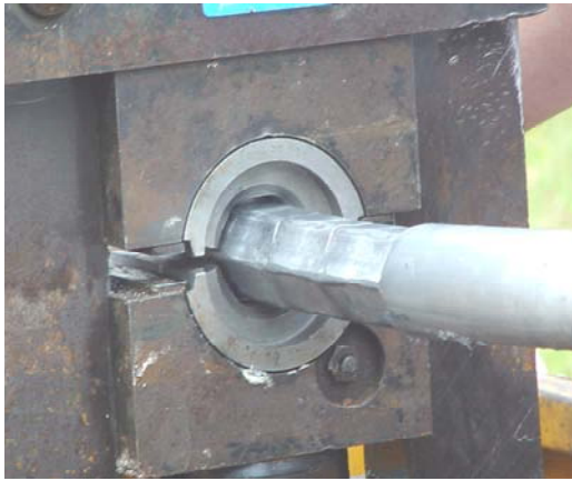
Figure 8- Installation of Alcoa compression splice.
