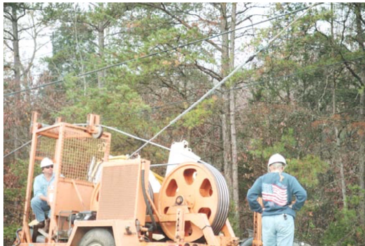
Figure 3- Bull wheel tension of conductor during installation
