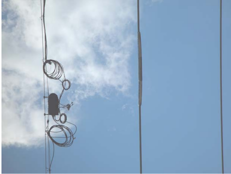
Figure 6 Thermocouples wiring for in-situ – temperature monitoring
