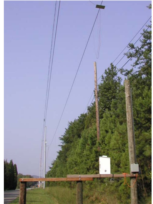
Laser at mid-span measure conductor sag
