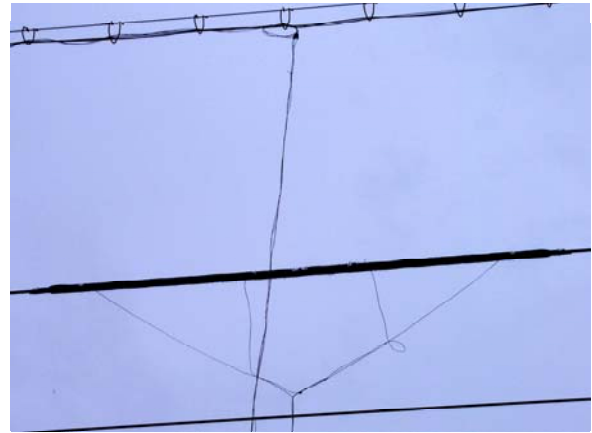
Figure 9- Installed PLP THERMOLIGN R Splice
