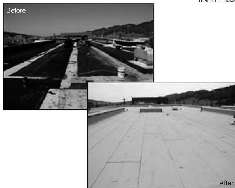
Fig. 4.12. Replacement of deteriorated roof on Building 9113 with a sustainable white roof.
