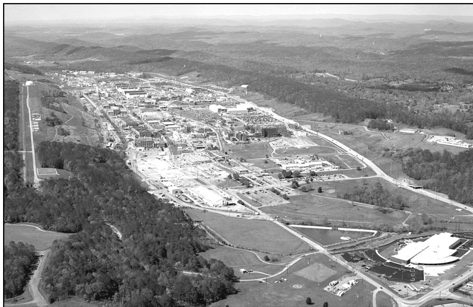
Fig. 1.8. Y-12 National Security Complex.
