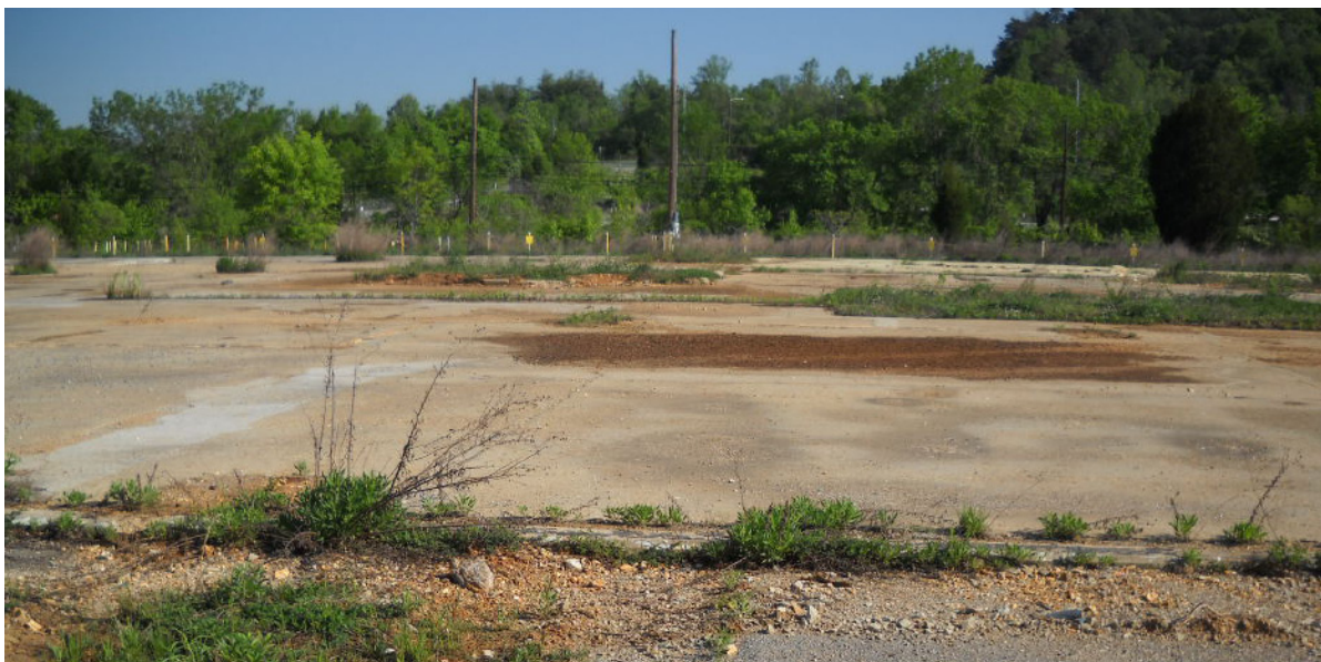
Fig. 3.18. The K-1420 pad after demolition.
