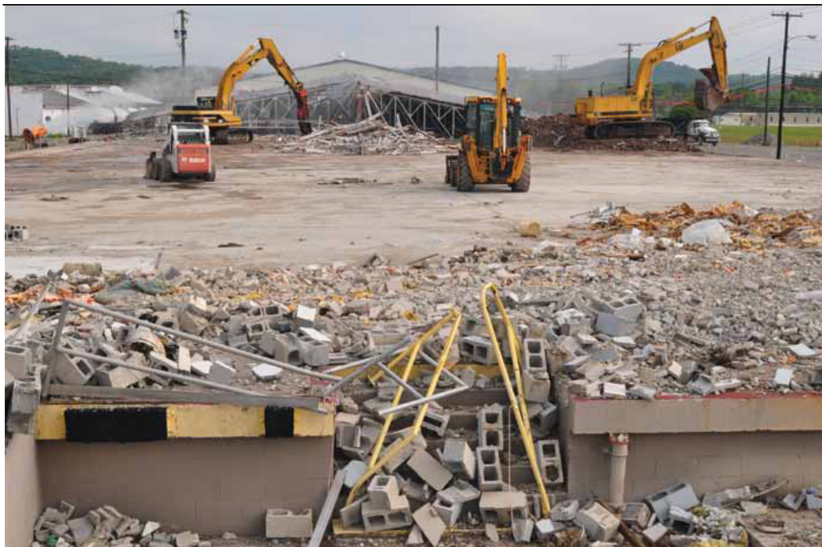
Fig. 3.23. K-1035 building demolition.
