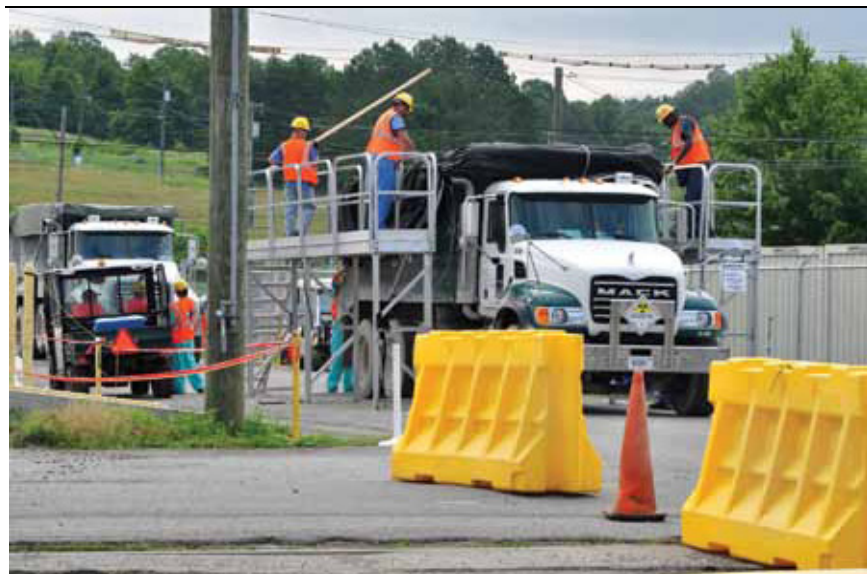
Fig. 3.24. Demolition debris generated from K-1035 building being sent to EMWMF.
