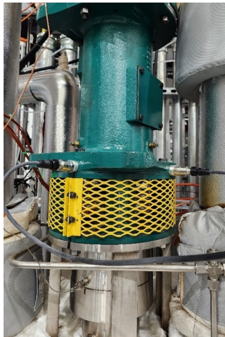
Figure 7. Locations of accelerometers on pump.
