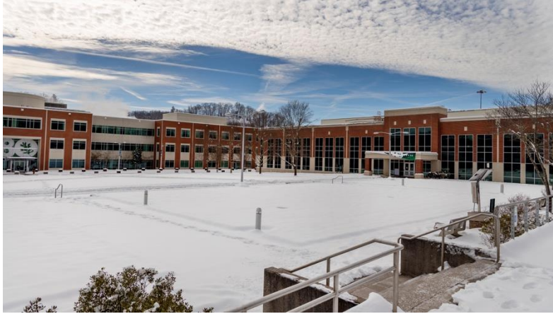
Figure 9. ORNL during January 2024 winter storm.
