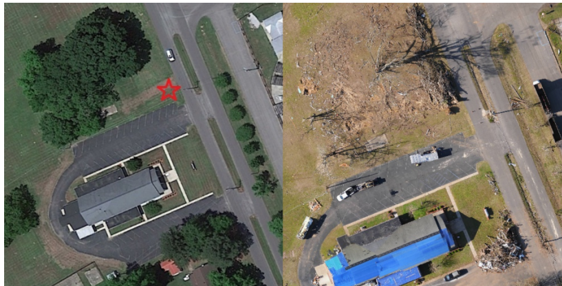
Figure 5. Location 1: Pre-storm (left), post-storm (right)
