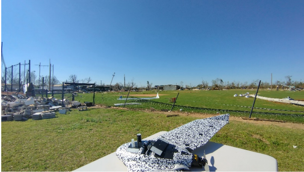
Figure 10. Damaged ball field at Location 2
