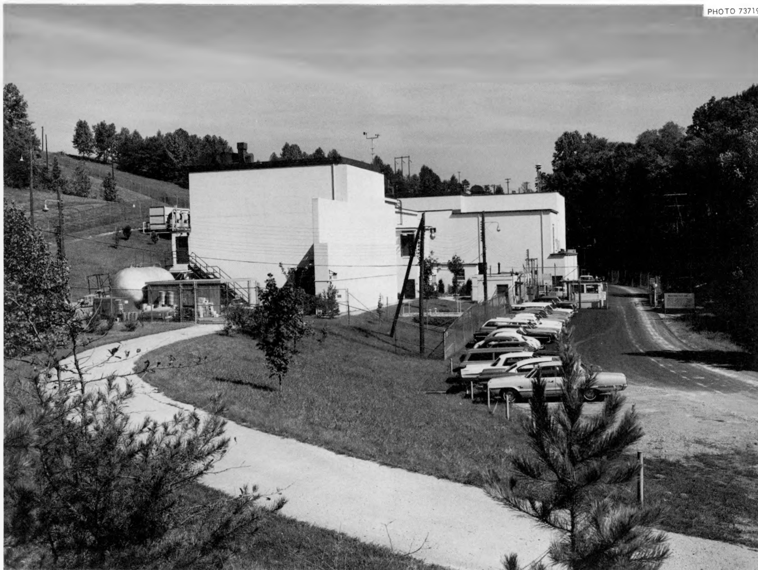
Fig. 3. West End of Building 9213 Showing the Concrete Shielding Wall Between the Roadway and the Large Doors.
