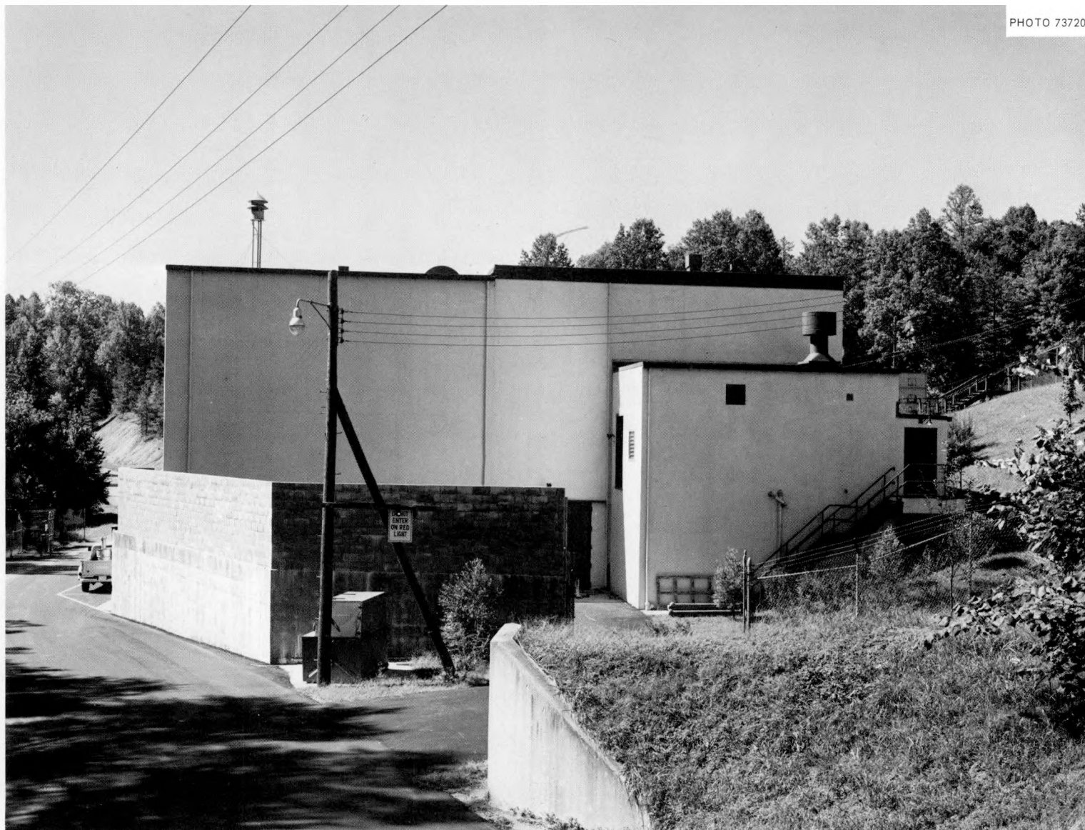
Fig. 4. East End of Building 9213 Showing the Concrete Walls and Bunkers which provide Shielding.
