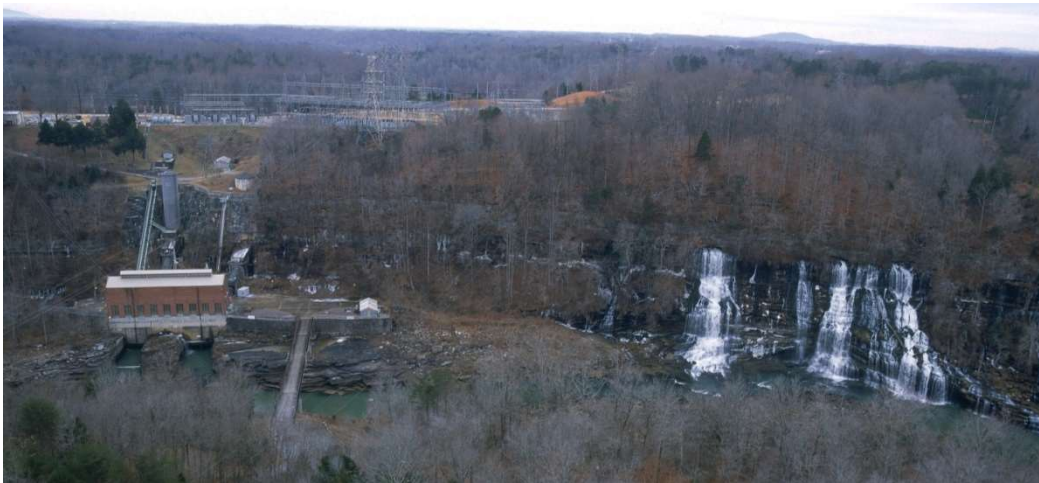
Figure 12. Great Falls leakage (Tennessee; powerhouse shown at left).
