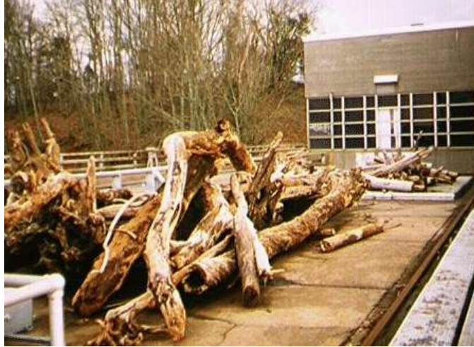
Figure 22. Debris removed from trash racks can range in size from aquatic milfoil to tree trunks. Shown by Jones et al. [2].
