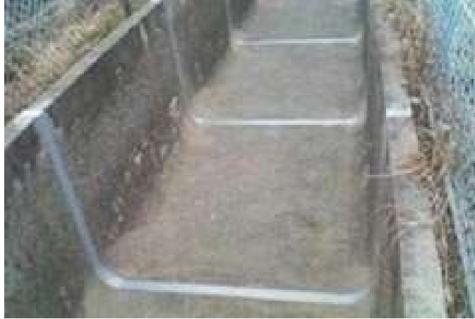
Figure 10. Waterstop repair in concrete channel.
