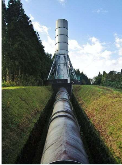
Figure 15. Steel surge tank at Isawa II Power Station (Japan).
