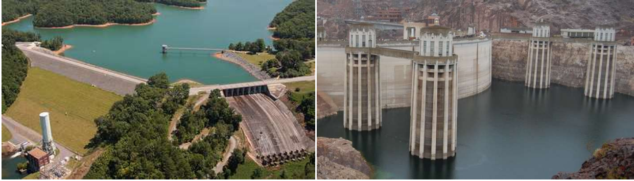
Figure 19. Tower intake structures. (left) Blue Ridge Dam (Fannin County, Georgia); (right) Hoover Dam (Clark County, Nevada/Mohave County, Arizona).
