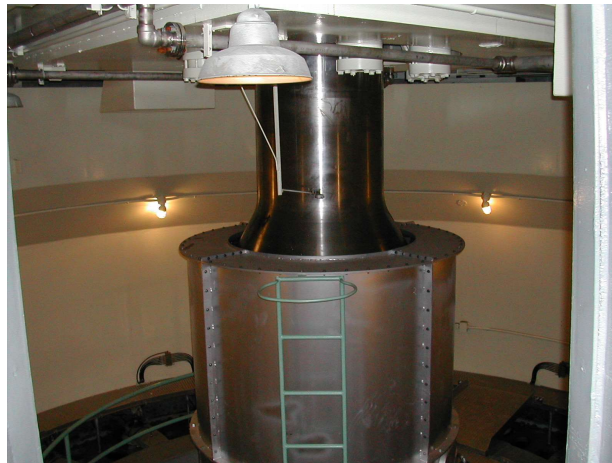
Figure 132. Turbine shaft/wheel pit.
