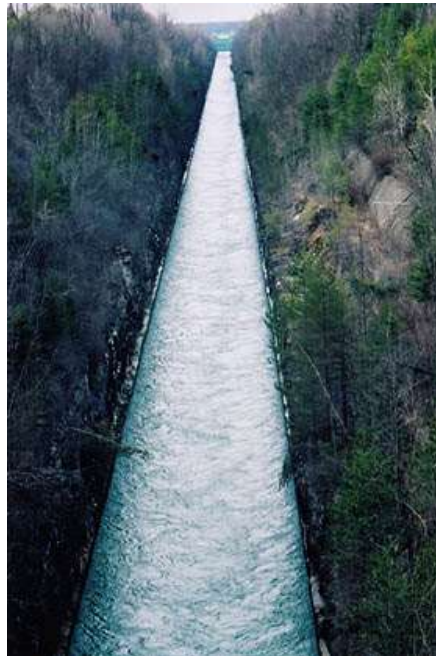
Figure 6. Open channel (Sir Adam Beck #1 Power Station, Niagara River, Canada).
