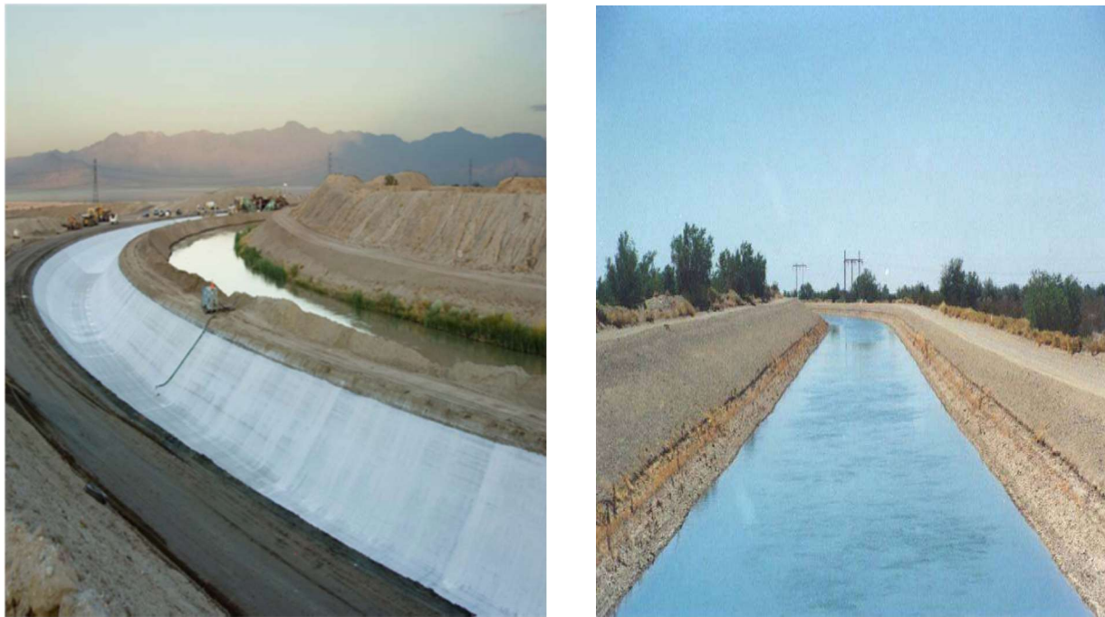
Figure 7. Coachella Canal concrete lining project (Coachella County, California).
