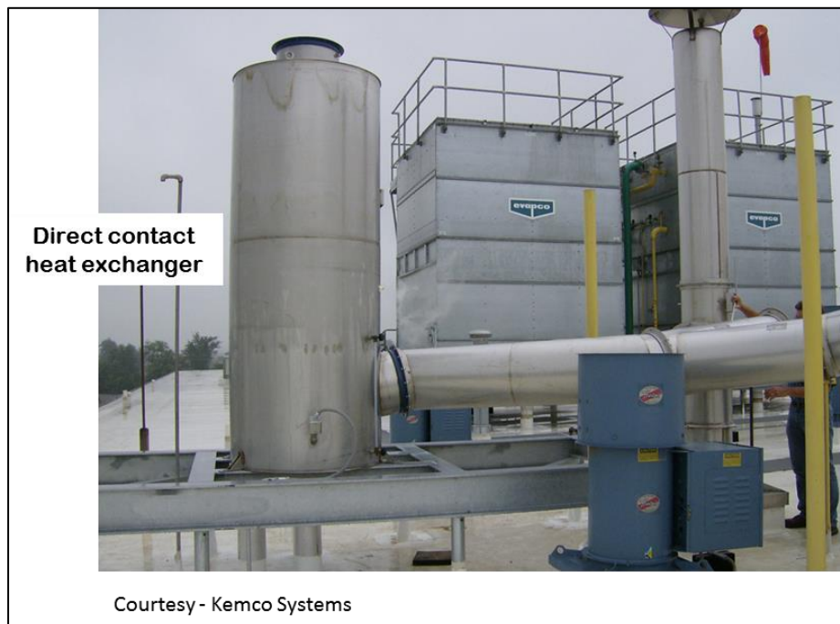
Figure 3-8. Installation of a direct contact condensing heat exchanger on a boiler.
