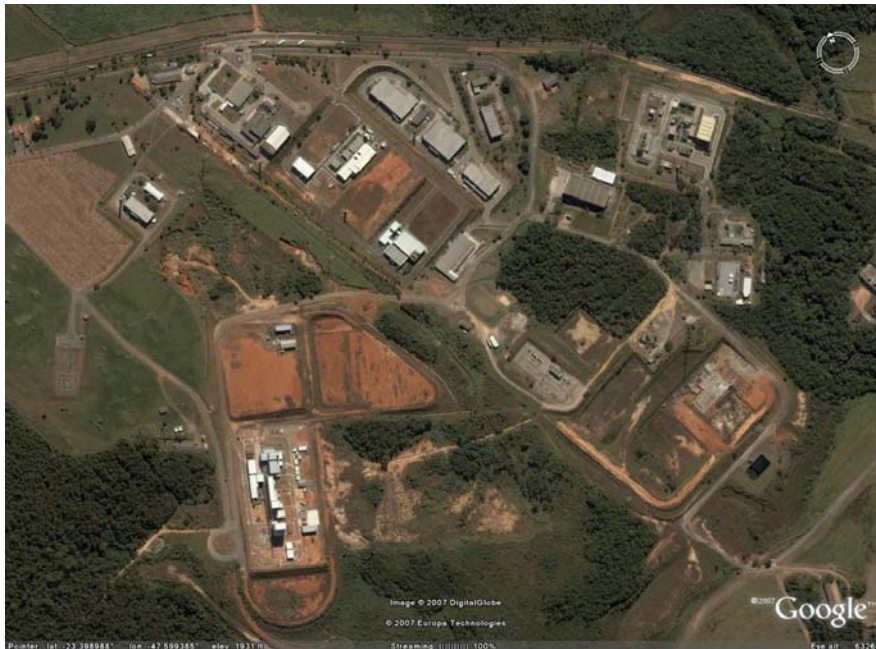
Fig. 24. Aramar Experimental Center, Brazil. Source: Google Earth
