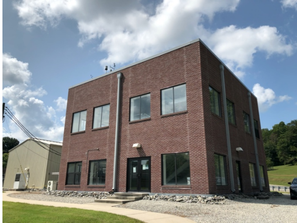
Figure 1. The ORNL FRP building on Bethel Valley Road. It is a two-story office building with five rooms on each floor. Meteorological monitoring is installed on the roof on which a MERV 7/8 filter pack is installed to provide central air.
