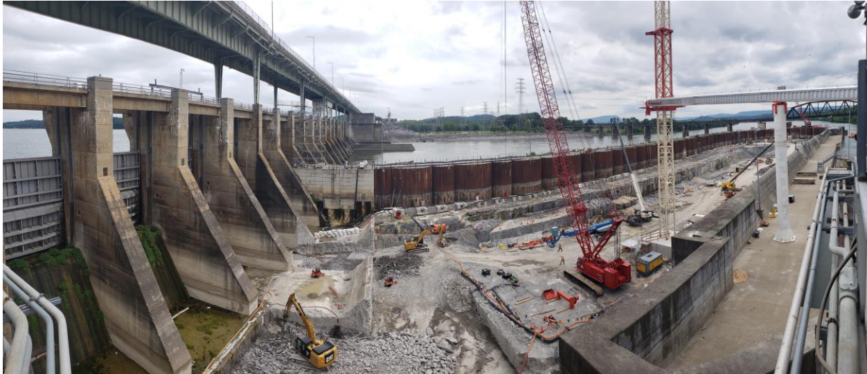
Figure 21. Chickamauga Lock replacement project 28 in Chattanooga, Tennessee, showing foundation excavation and treatment within the dewatered/coffer dammed work site. Image courtesy of Scott DeNeale.
