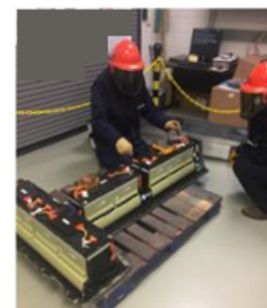
11) Measure Internal Voltages
