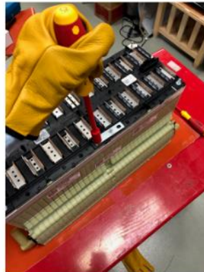
5) Remove (4) 10mm nuts that connects two 46 V modules together by bus bar.
