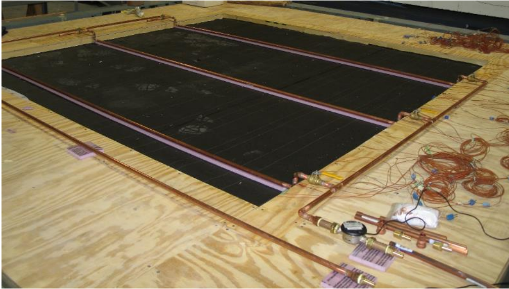
Figure 5. Copper tubes (3) with circulating water used as heat sink or source.
