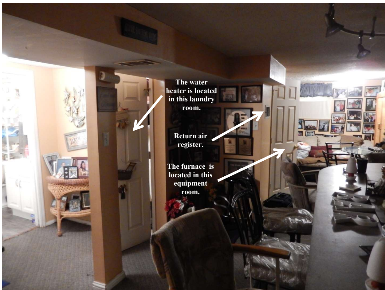
Figure 5.18. Basement equipment rooms in House MO3.
