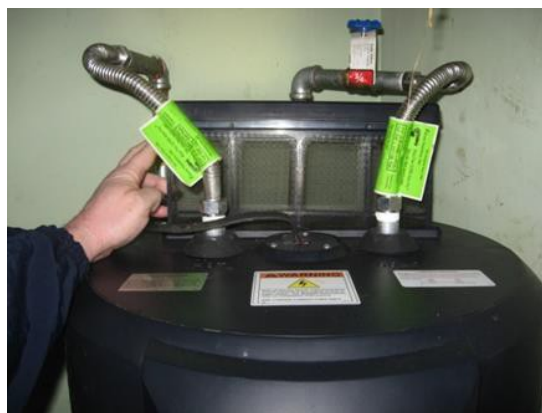
Figure 4.14. GE heat pump water heater filter.
