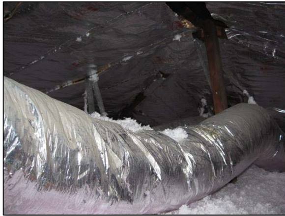
Figure 4.24. Radiant barrier installed on rafters, ridge vent, and additional blown-in insulation installed.
