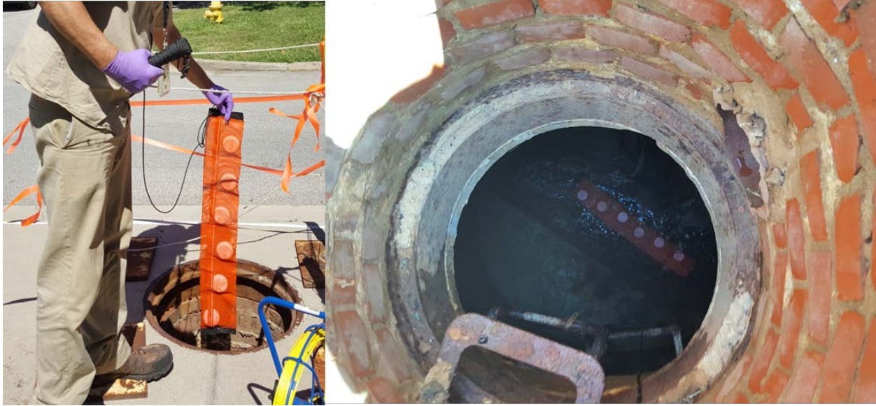
Figure 3-2. Deployment of ascorbic acid tablets in mesh bags into Manhole MH211-3.
