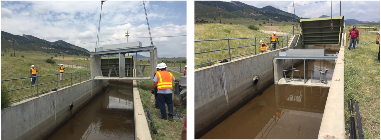
Fig. 8. First set of casted parts being installed in the Denver pilot.
