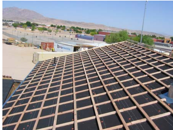
Figure 5. Double batten system installed on Units N4 and N8.
