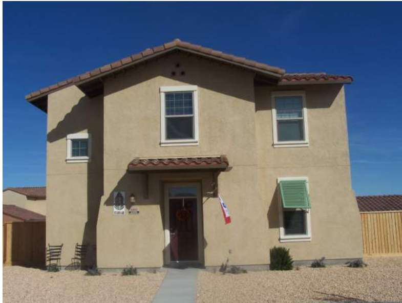
House N10 has concrete tile nailed direct to deck. The tile have conventional paint pigments. The front door of house N10 is facing west.
