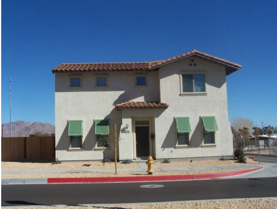
House N4 has concrete tile placed on double battens. The tile are coated with Cool Tile IR COATING™. The front door of house N4 is facing west.
