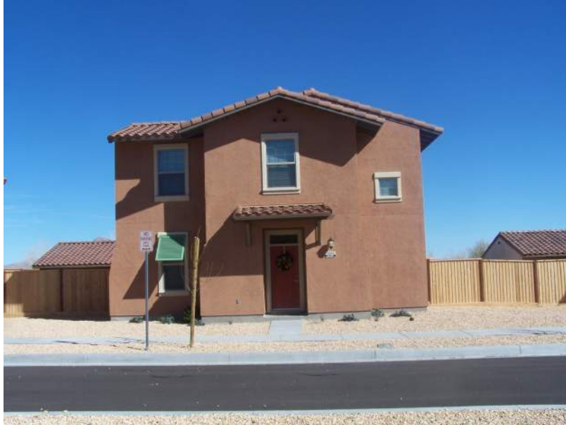
House N5 has concrete tile nailed direct to the deck. The tile are coated with Cool Tile IR COATING™. The front door of house N5 is facing west.
