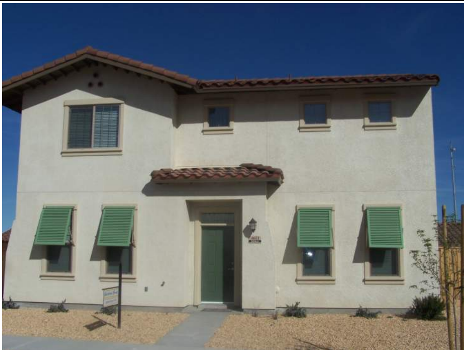
House N8 has concrete tile placed on double battens. The tile have conventional paint pigments. The front door of house N8 is facing west.
