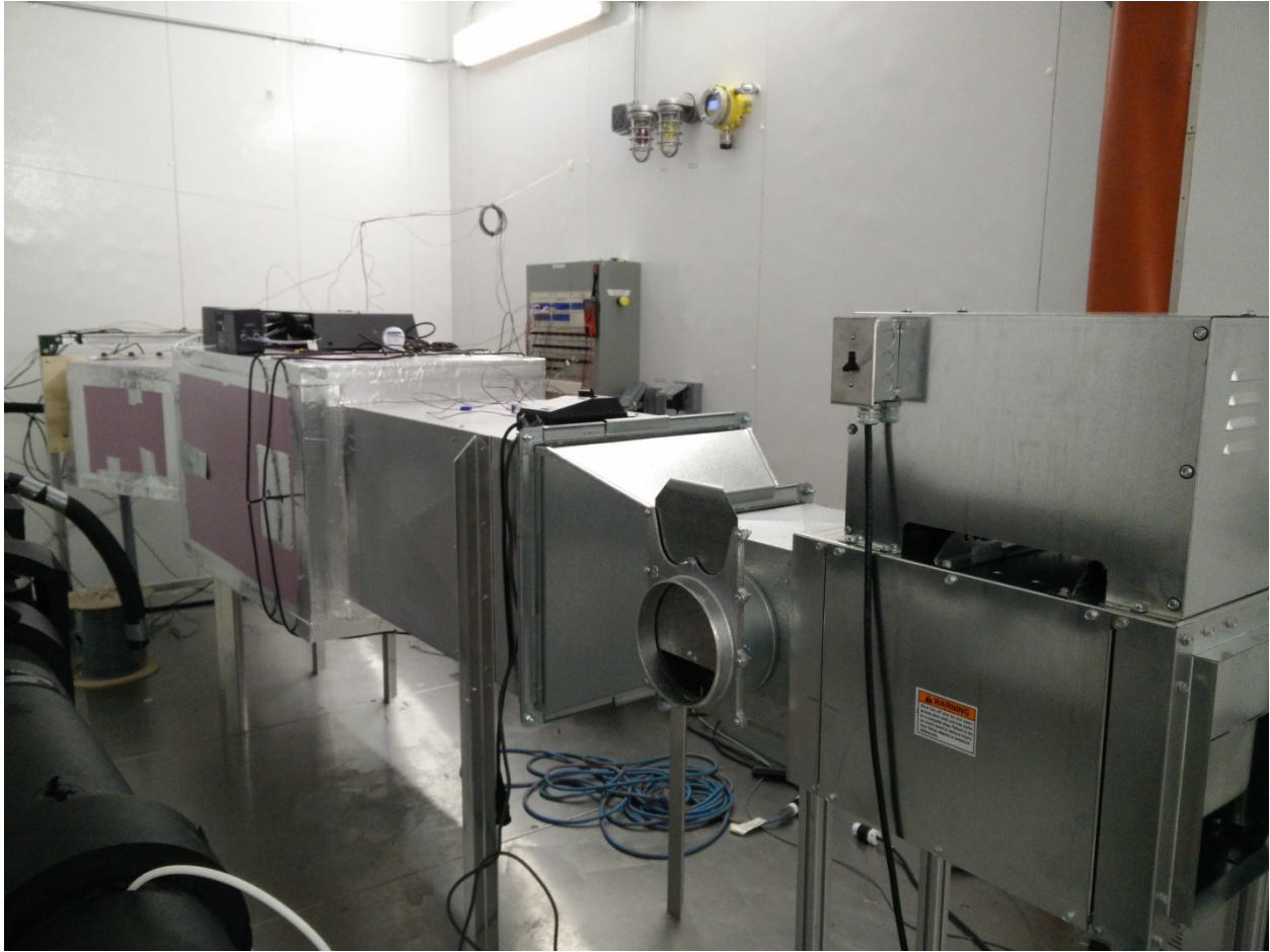
Figure D.4. Indoor air enthalpy tunnel fully instrumented and connected to the data acquisition system.
