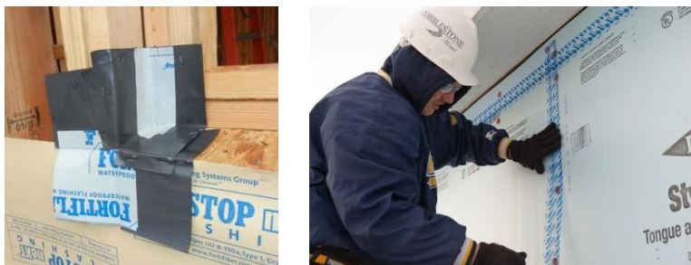
Figure 1. Tape used to flash window rough openings (left) and to seal joints between boards (right).
