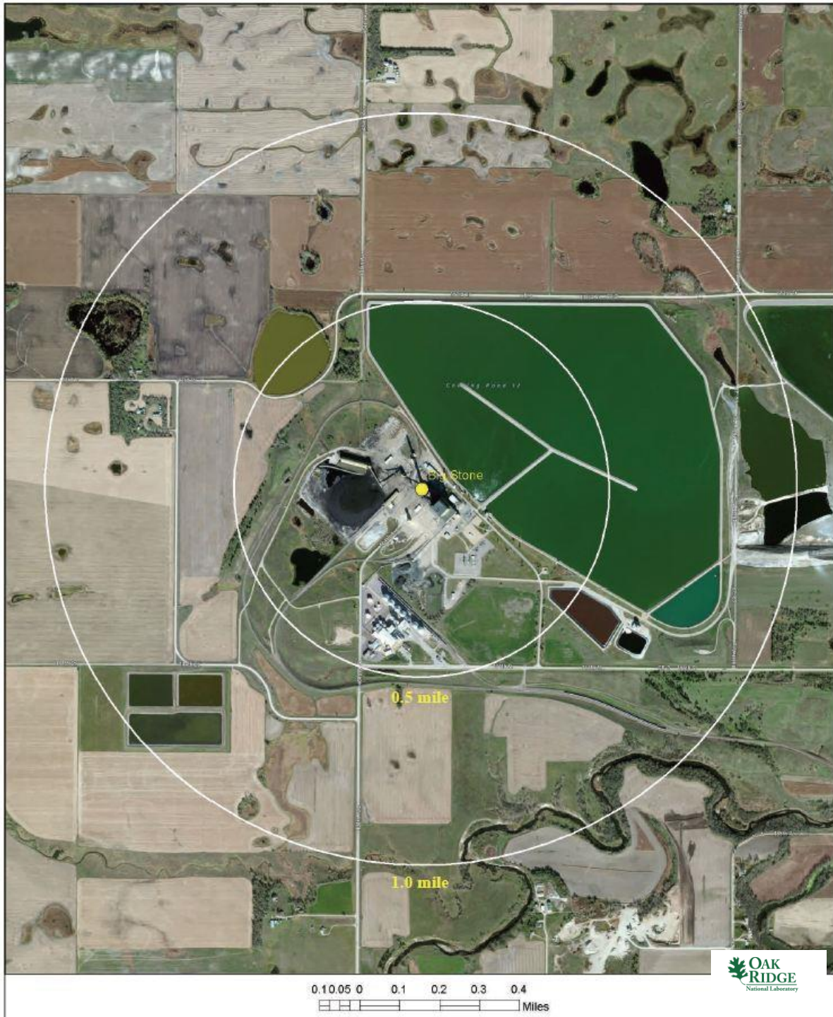
Fig. A.21. Satellite view of Big Stone Power Plant proximity.
