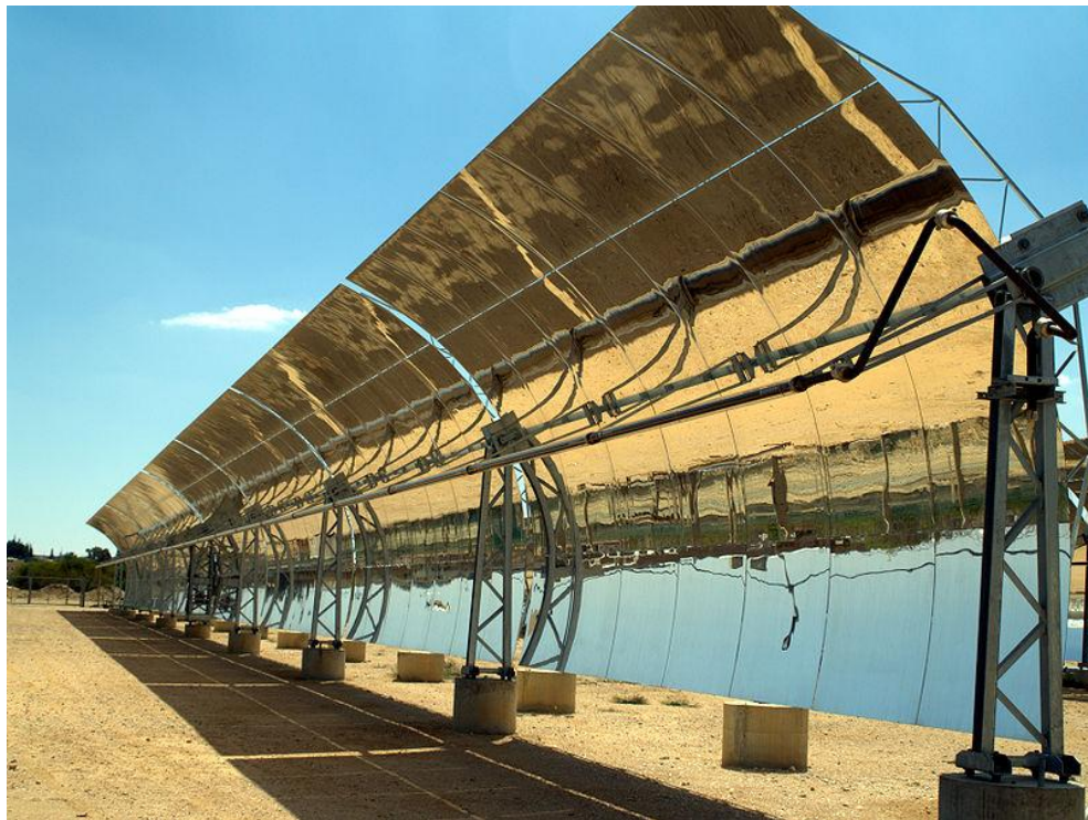
Figure 1) Solar Trough Plant, located in Beersheba, Israel
