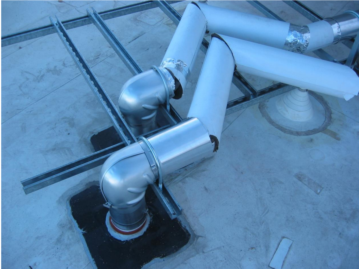
Figure 9) Insulated fluid line penetrations.
