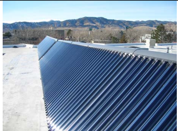
Fig. 14.b. Solar roof vacuum tubes
