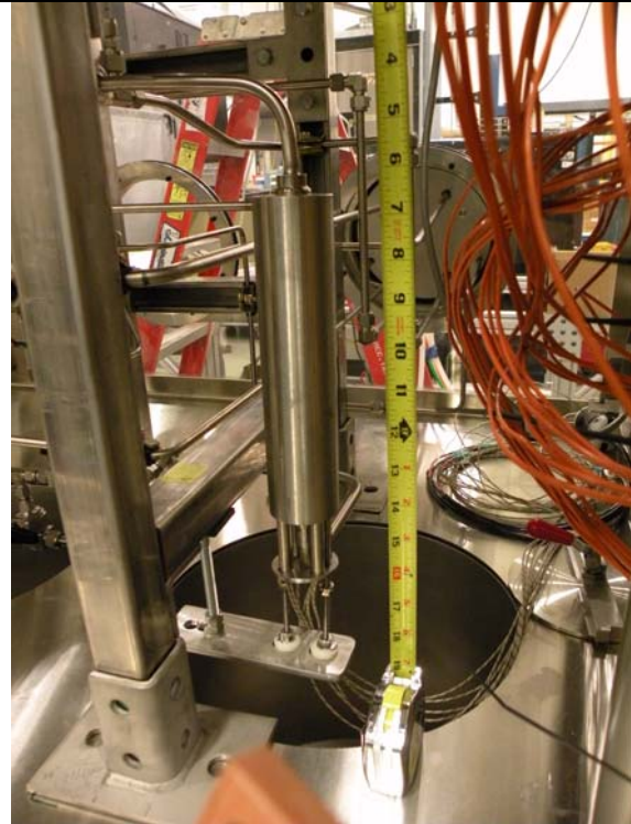
Fig. 9b. 2.4 kW heater before insulating.
