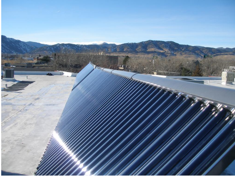
Figure 6) Completed solar collector field.
