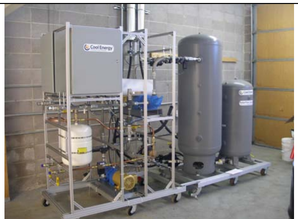
Fig. 14d. Solar storage tank and thermal expansion tank before installation.
