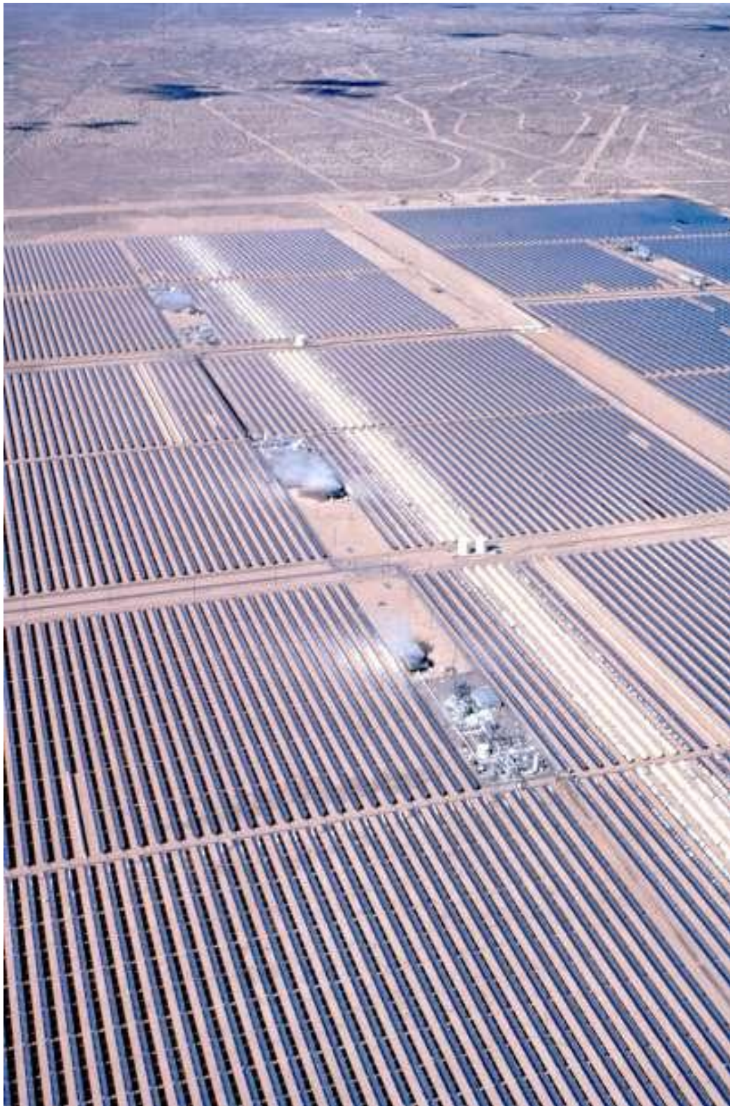
Figure 30) SEGS III through VII projects, Kramer Junction, California
