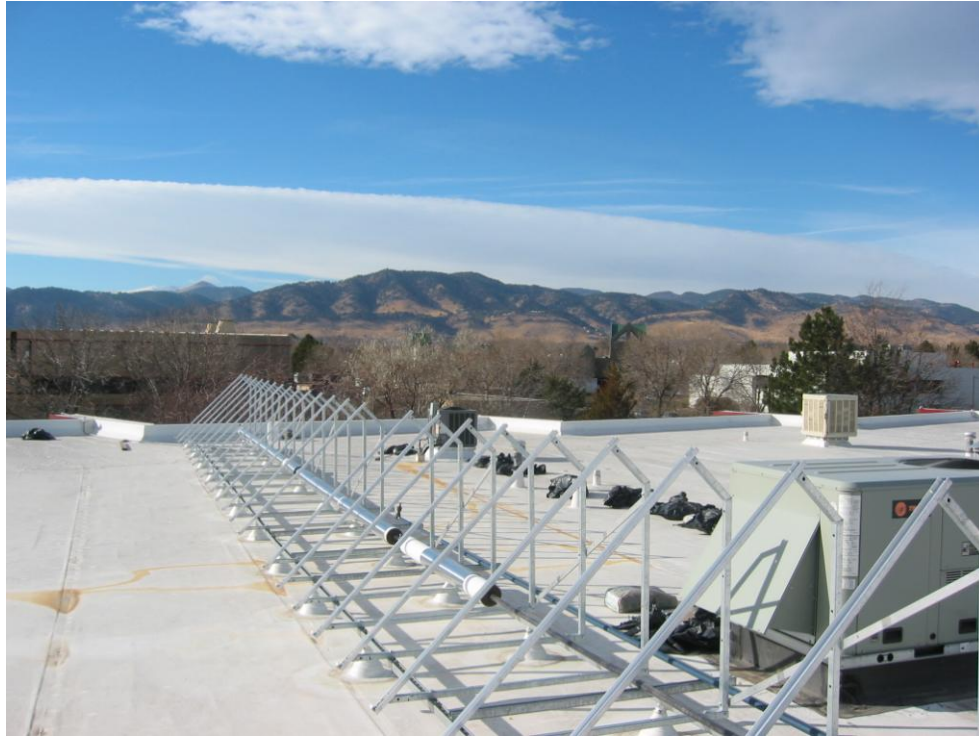
Figure 4) 45° tilt angle rack assembly installed.
