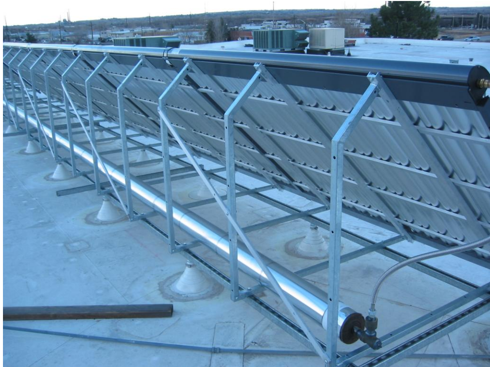
Figure 5) Solar collectors installed on rack assembly.
