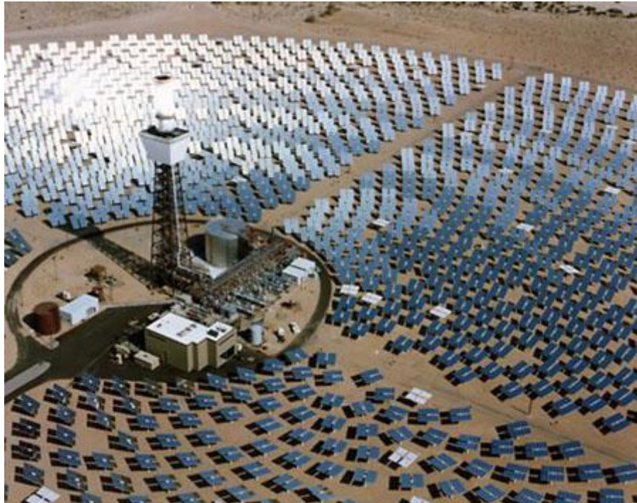
Figure 2) Solar One/Two Power Tower Facility, near Dagget, CA
