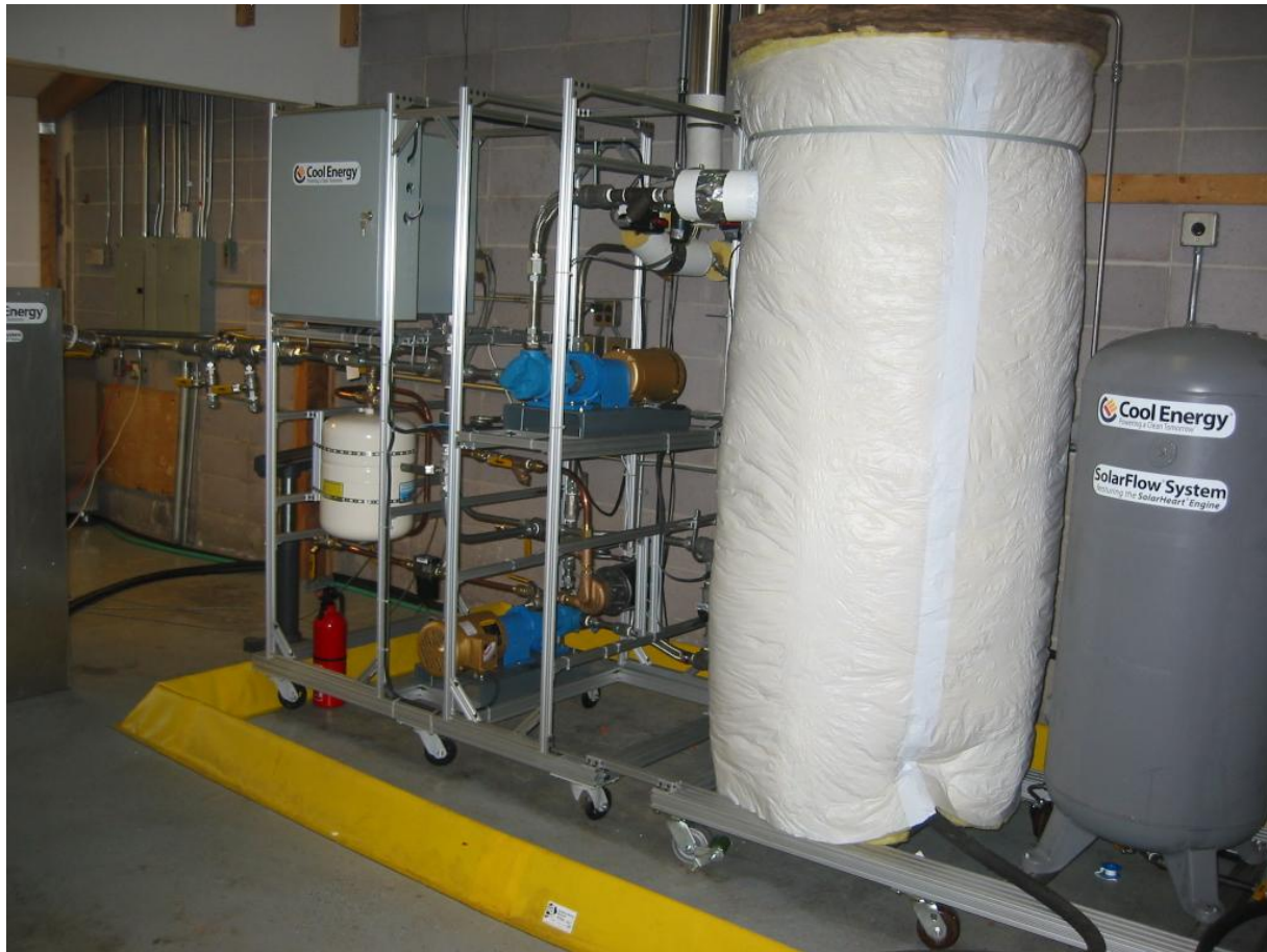
Figure 14) Equipment skid with tank insulation operating on solar thermal energy from solar field.
