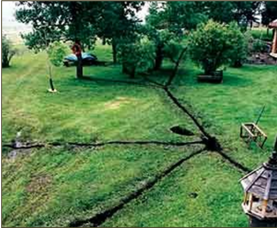
Fig. 9. Hydro-vacuum excavation method used to dig a slot trench.
