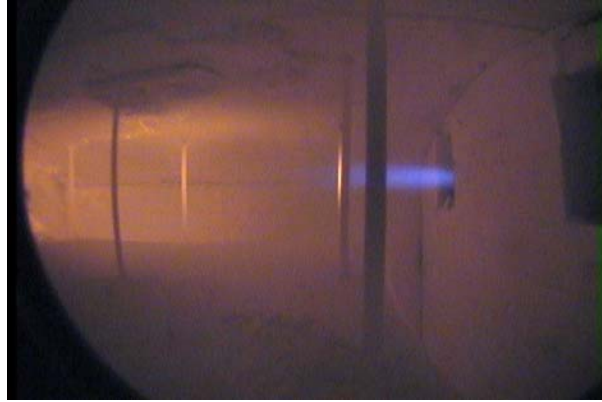
Figure 1. Upper chamber of the furnace as viewed by the FIA camera
