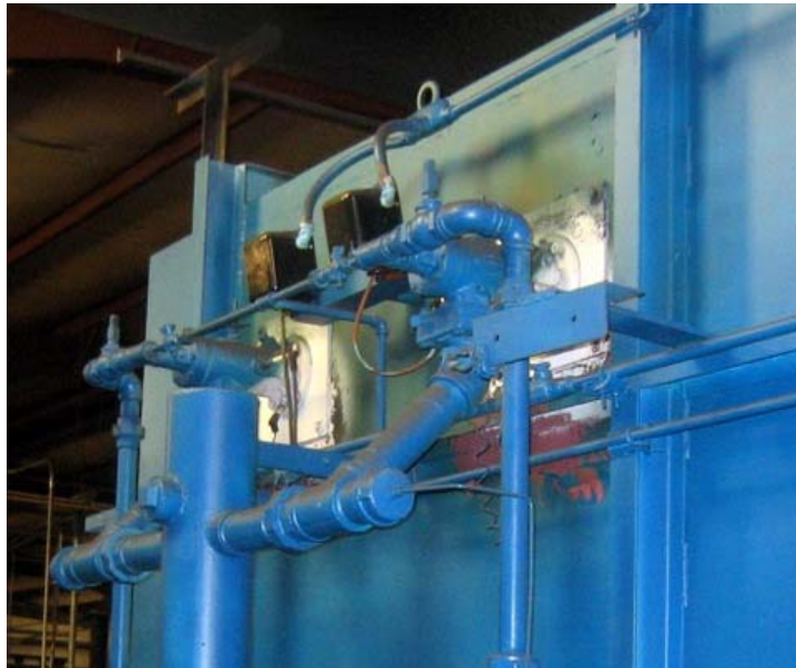
Figure 2. View of Eclipse burners installed in heat treating furnace.
