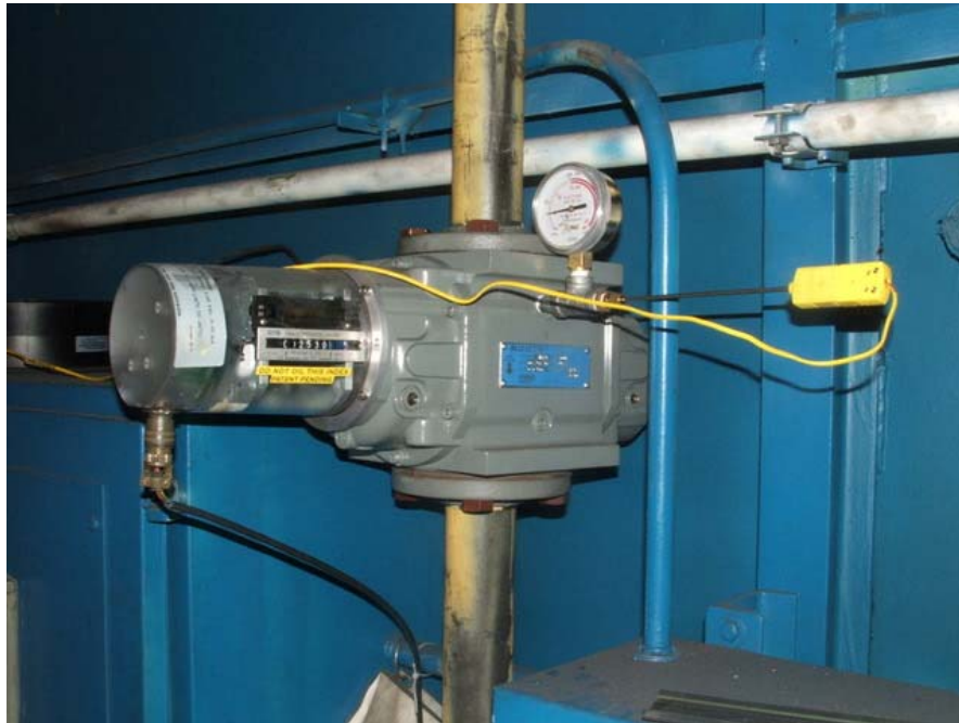
Figure 4. Fuel volume flow, pressure and temperature instrumentation installed on furnace gas
