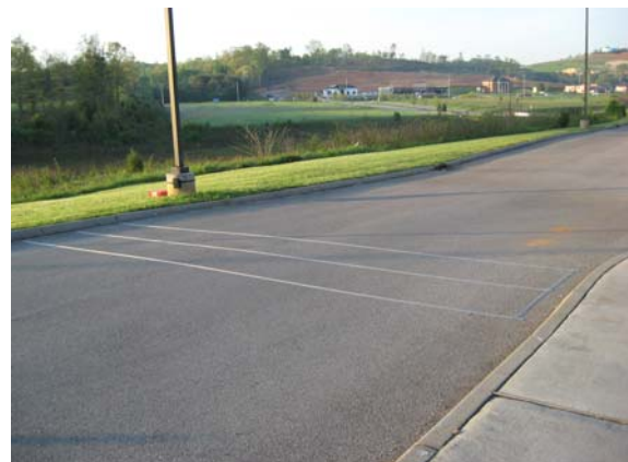
Figure 23 Tennessee FOT Deployed Prototype Sensor 2(ORNL 2) and GT Infrared Sensor 2
