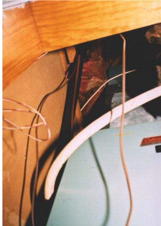
Figure 3.2. Unsealed equipment chase permits infiltration.
