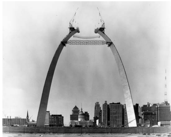
Figure 47: Construction of the St. Louis Arch
