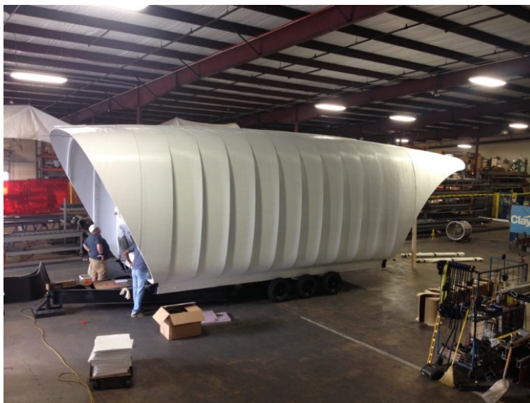
Figure 35: ORNL AMIE structure
