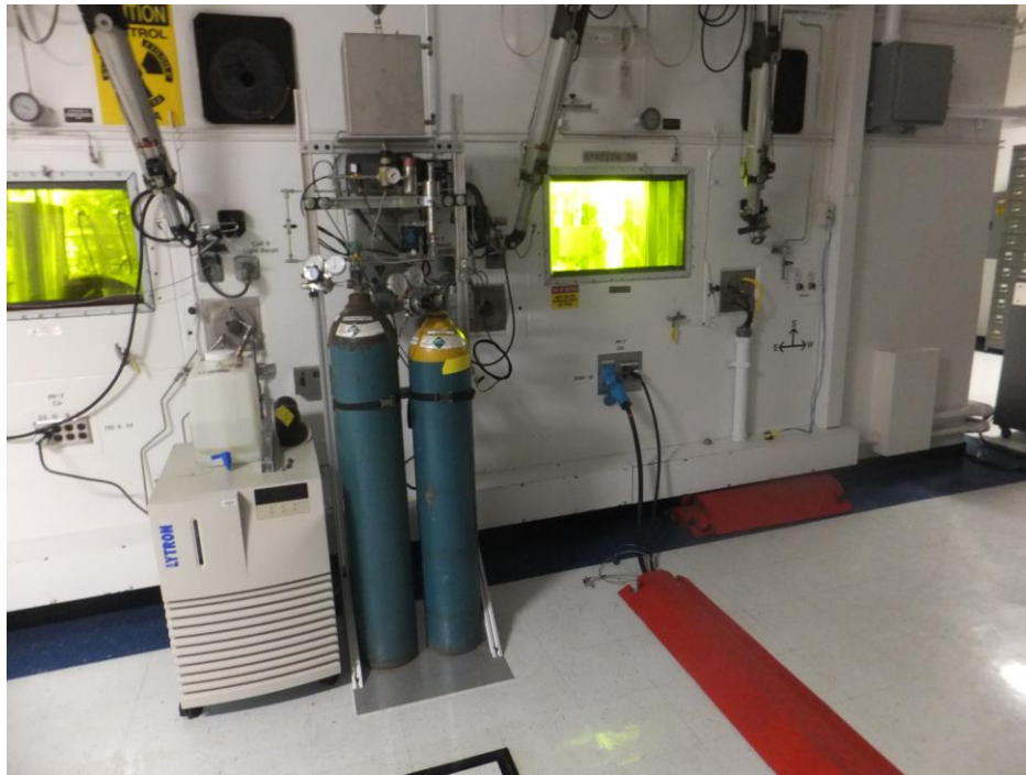
Figure 17. Water cooling system and high-pressure system for the in-cell LOCA apparatus.
