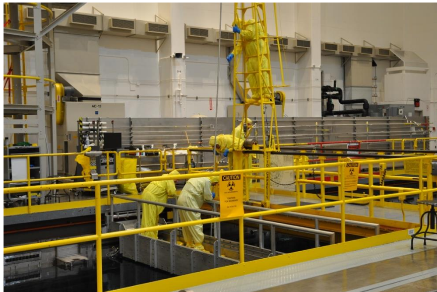
Figure 15. The irradiation chamber was lowered down into the spent fuel element.
