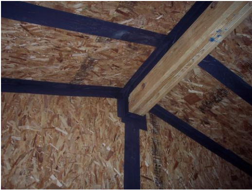
Figure 26. Peel-and-stick panel tape provides added assurance that panel seams will remain airtight.
