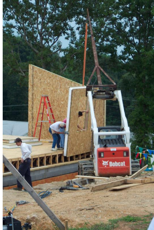
Figure 42. Mounting the wall panels on the side of the floor trusses leaves easy access to run electric wires from the walkout lower level into the vertical wiring chases in the wall studs.
