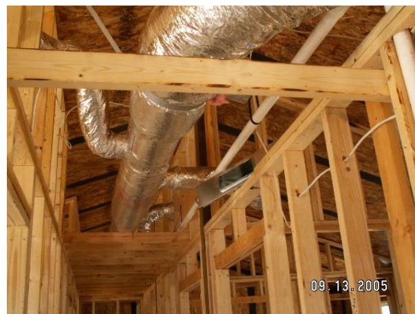
Figure 36. Supply ducts located in the conditioned chase formed by the ceiling SIPS and dropped ceiling.
