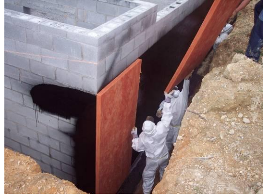
Figure 22. Installation of 4 x 8-ft fiberglass boards sized to cover the waterproofing.
