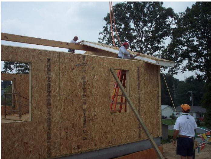
Figure 32. The SIP roof panel installation.
