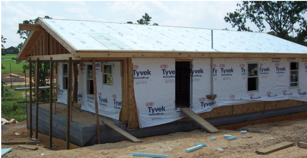
Figure 5. Two inches of XPS is laid directly on top of the 8-in.-thick SIP roof panels.
