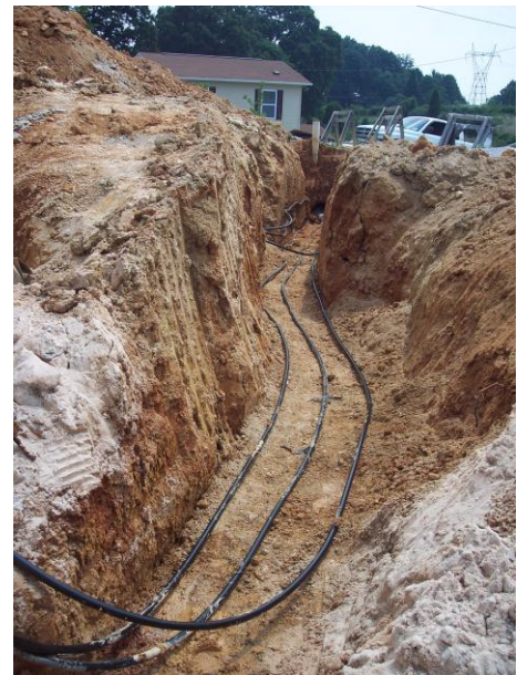
Figure 34. Geothermal heat exchanger pipe being installed in the trench dug for sewer lines.
