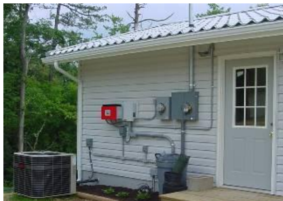
Figure 48. Sunny Boy (red box at left) installed in TVA-approved Green Power Generation hookup.
