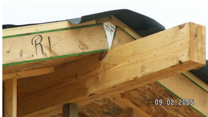
Figure 41. A wedge of foam is provided by the SIP manufacturer to fill the space at the ridge.
