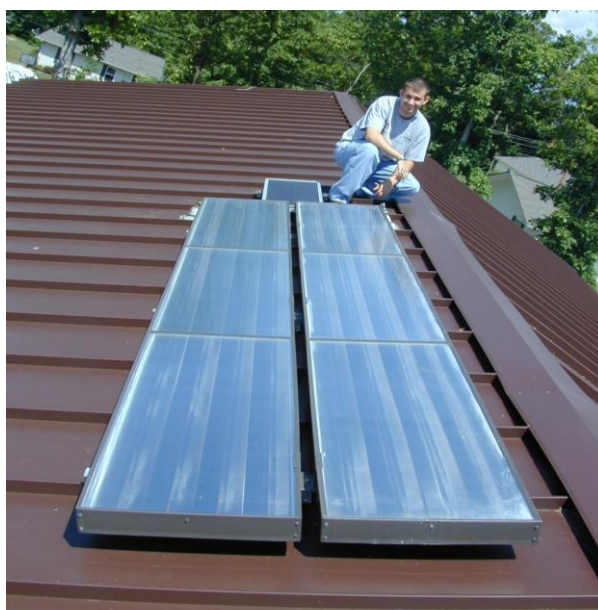
Figure 49. SolarRoofs, SkyLine System 5 solar water heater, with 38 ft 2 of solar collector area installed on the roof of ZEH5.
