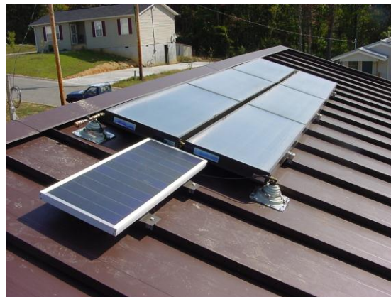
Figure 6. Solar water heater collectors.
