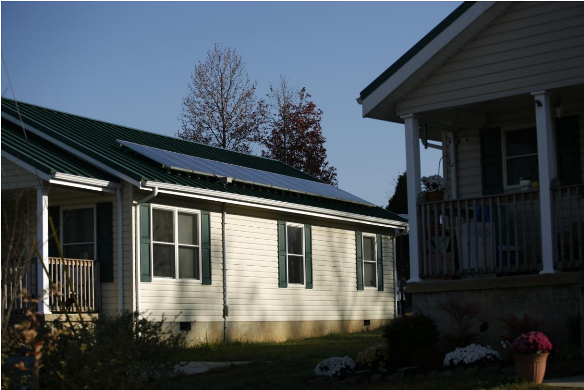
Figure 45. Solar modules sit nicely on the roof of ZEH2. The dark green roof makes for a very pleasing appearance with the dark bluish-green polycrystalline module.
