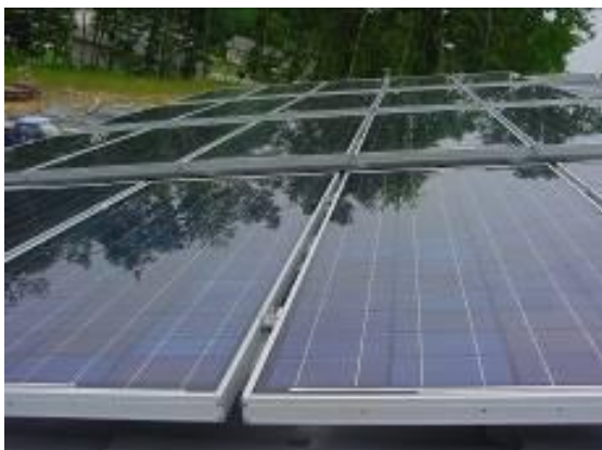
Figure 47. PV modules are clamped to aluminum rails and carefully grounded.
