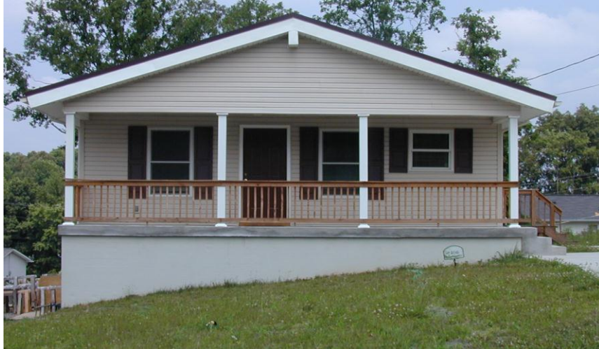
Figure 3. Picture of east elevation of ZEH5 from the street.
